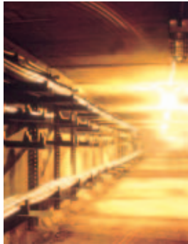
Installation in the Culvert
