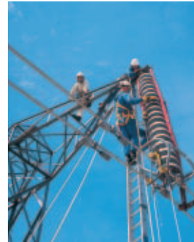
Overhead Transmission Line Project
