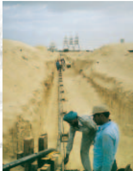
Underground Transmission Line Project
