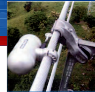
Vibration measurement on erected line
